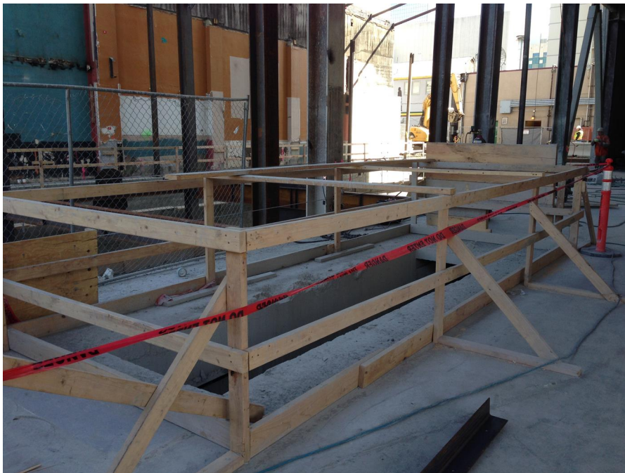
(Correct way to protect others at a floor penetration)
